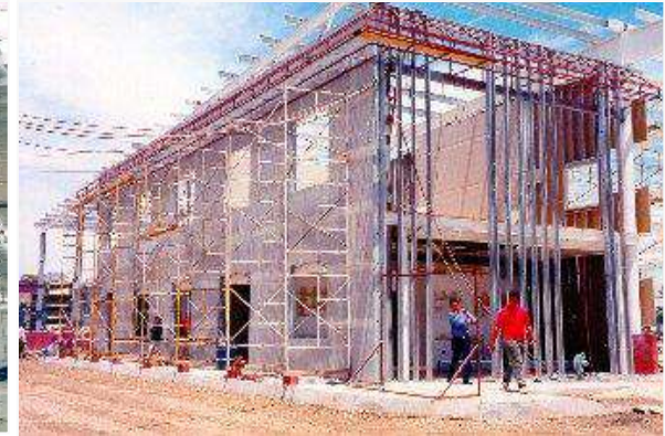
Nave Industrial "SKB" Maran
