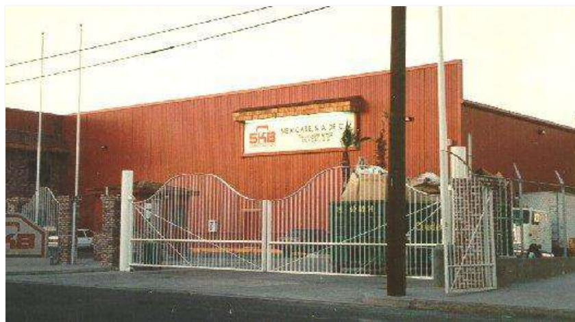
Nave Industrial "SKB" Maran
